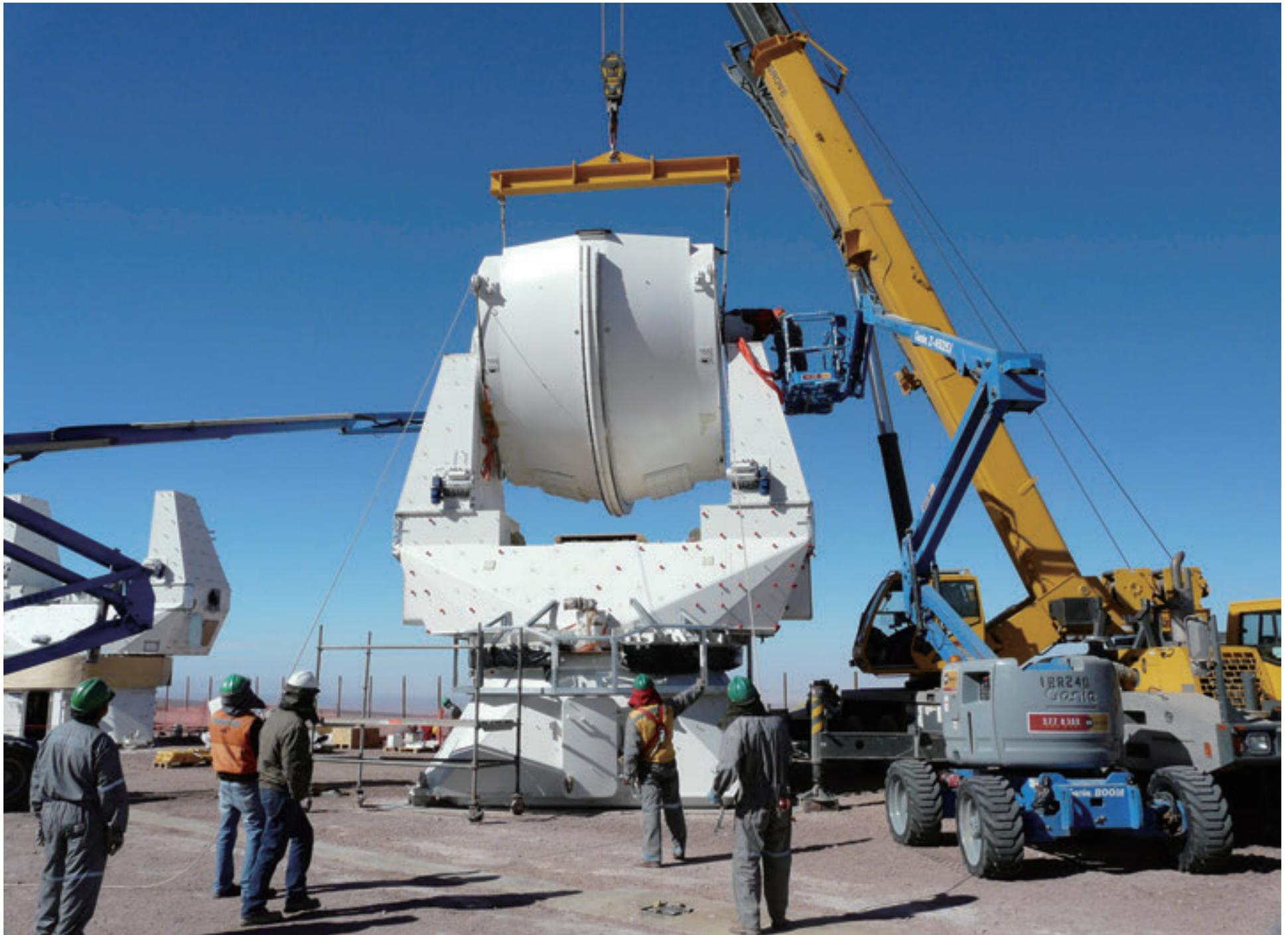
Assembling the receiver cabin on a European 12-meter antenna at the OSF. Credit: ALMA (ESO/NAOJ/NRAO)/S. Stanghellini (ESO)
