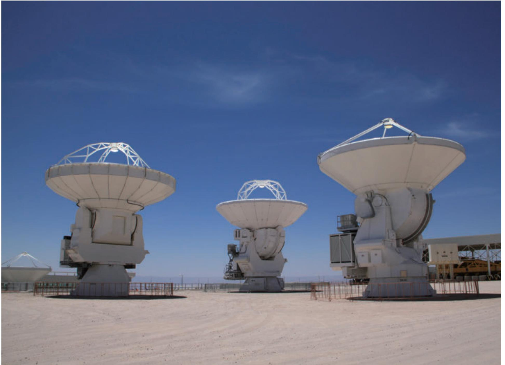
Three 12-meter antennas with a different shape at the OSF, constructed by North American, Japanese, and European partners (from left to right). Credit: ALMA (ESO/NAOJ/NRAO), M. Hiramatsu (NAOJ)
