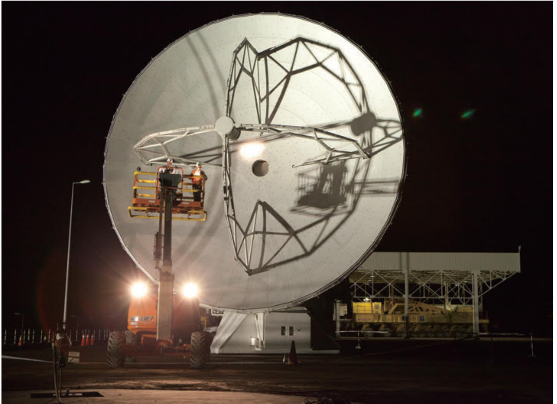
Inspection of the antenna surface at the OSF. Credit: ALMA (ESO/NAOJ/NRAO)
