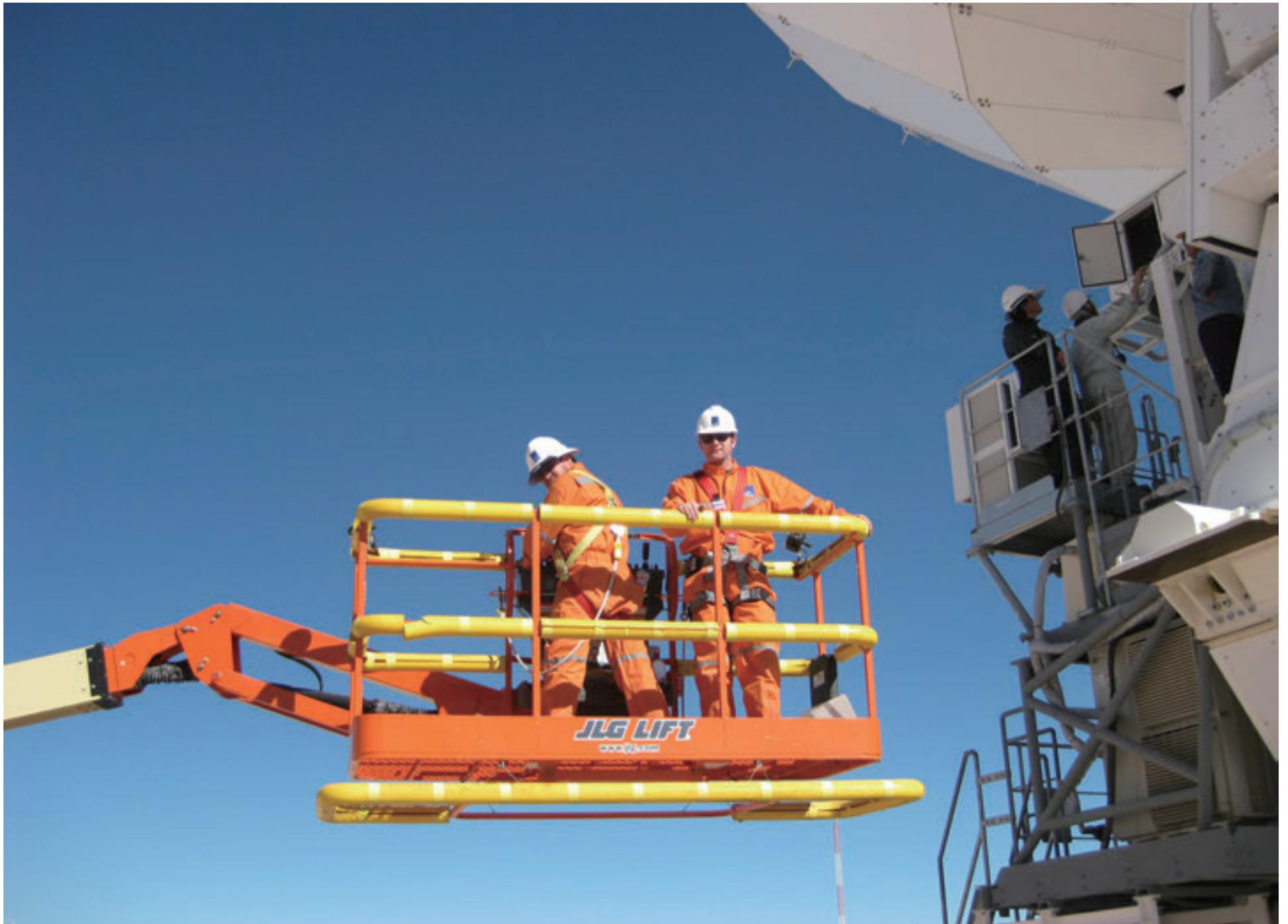
Maintenance work on an ALMA antenna at the OSF. Credit: ALMA (ESO/NAOJ/NRAO)
