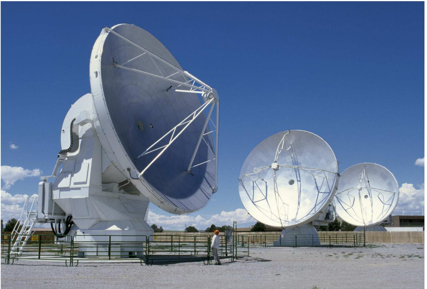
Figure 9: The Three Prototype Antennas at the ALMA Test Facility in Socorro
